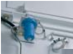
Leakage detector and cooling air temperature detector
